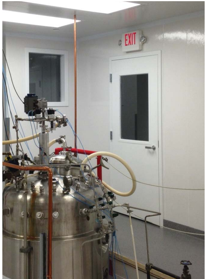
Panels were installed within 5 working days
