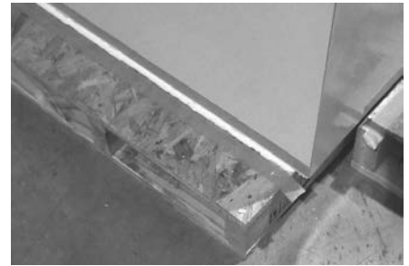
FIGURE 22: HORIZONTAL SEAM FILLED COMPLETELY WITH SEALANT
