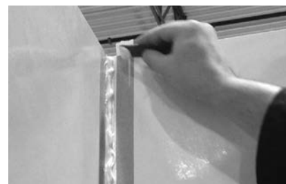
FIGURE 21: USING RADIAL SEAM FINISHER FOR ROUNDER CORNER JOINT
