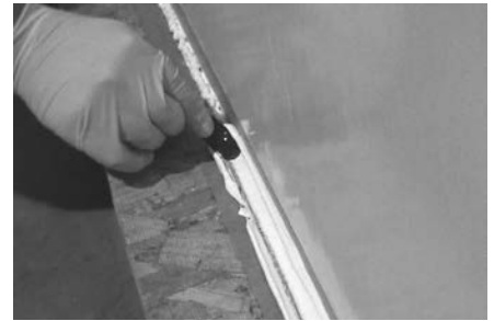
FIGURE 23: HORIZONTAL FINISH WITH ROUNDED CORNER
