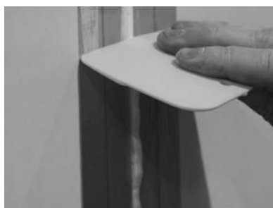
FIGURE 18: REMOVING EXCESS SEALANT
