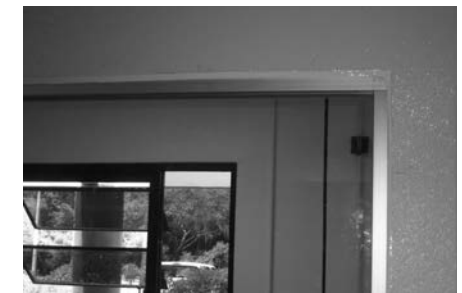
FIGURE 24: TYPICAL WINDOW SEAM APPLICATION
