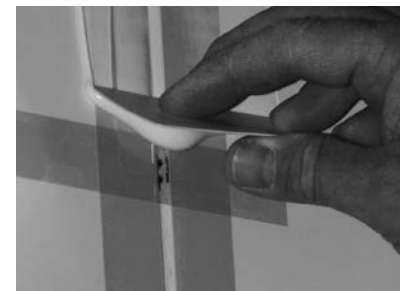
FIGURE 17: APPLYING THE PAINTER TAPE HORIZONTAL IN 3' SECTIONS
