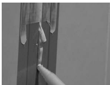
FIGURE 19: BUMP ADHESIVE IN TO PREVIOUS SECTION
