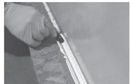
FIGURE 23: HORIZONTAL FINISH WITH ROUNDED CORNER
