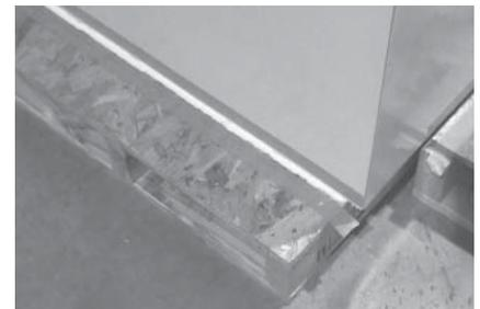
FIGURE 22: HORIZONTAL SEAM FILLED COMPLETELY WITH SEALANT
