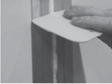
FIGURE 18: REMOVING EXCESS SEALANT
