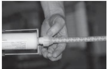
FIGURE 14: ATTACH STATIC MIXING TIP
