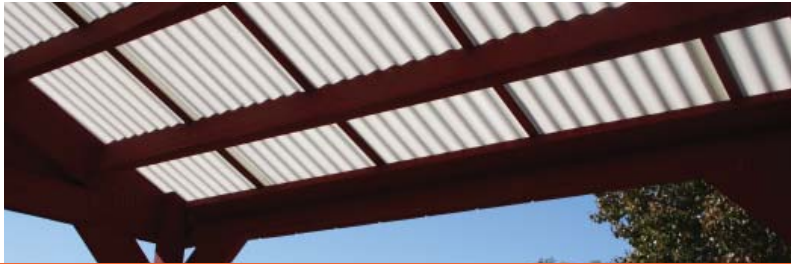
corrugated roofing panel installation
