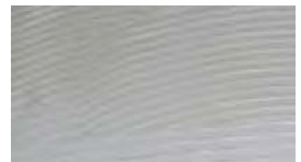
FIGURE 8: EXAMPLES OF PROPERLY TROWELED ADHESIVE APPLICATION
