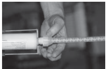
FIGURE 14: ATTACH STATIC MIXING TIP
