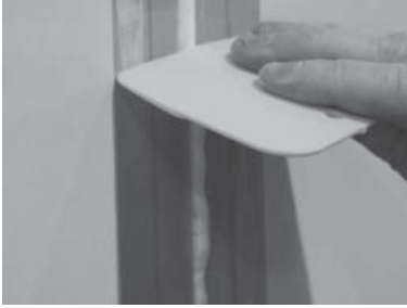
FIGURE 18: REMOVING EXCESS SEALANT
