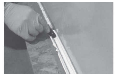
FIGURE 23: HORIZONTAL FINISH WITH ROUNDED CORNER
