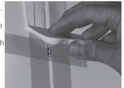
FIGURE 17: APPLYING THE PAINTER TAPE HORIZONTAL IN 3' SECTIONS
