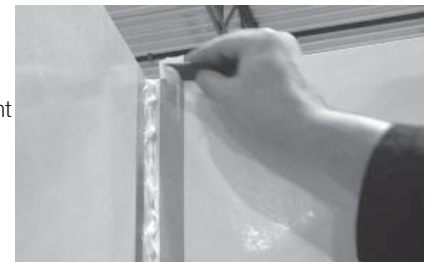
FIGURE 21: USING RADIAL SEAM FINISHER FOR THE SEAM. REMOVE ANY EXCESS SEALANT
