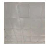
When FRP panels are placed in the grid, there will be a space due to the design of the grid. This space is accented, when using smooth panels.
