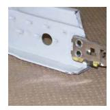
Using heavy duty grids with lip and flange (pictured above), may result in a space when FRP panels are installed in the grid. (see photos below).
